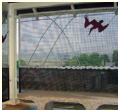
44 Fast Food • 2003 Schmidt Design Group Bus Shelter, Silver Strand Hwy. at Loews Coronado Bay Rd.
