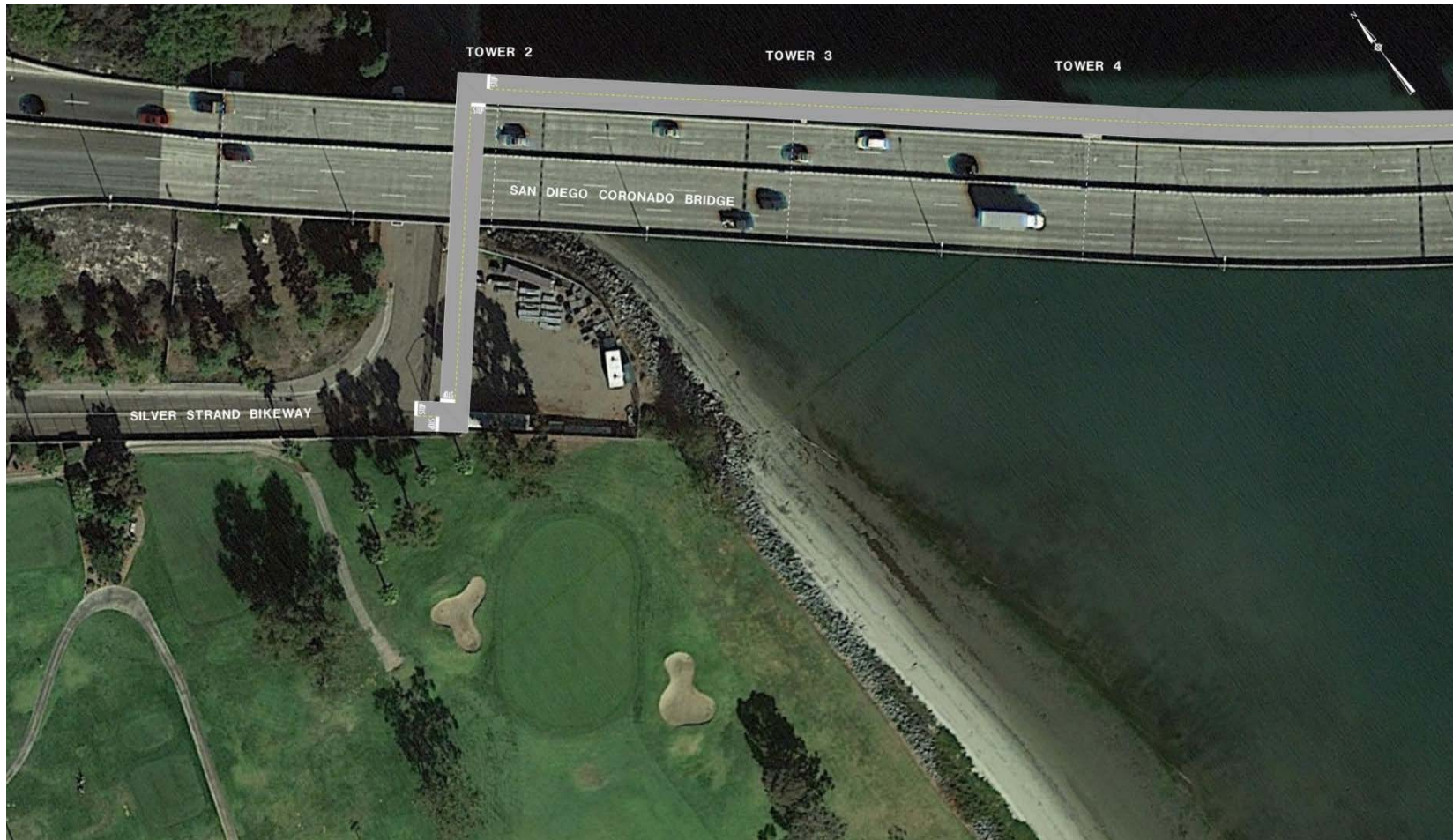
Figure 12 – Caltrans Maintenance Yard Connection Aerial View
