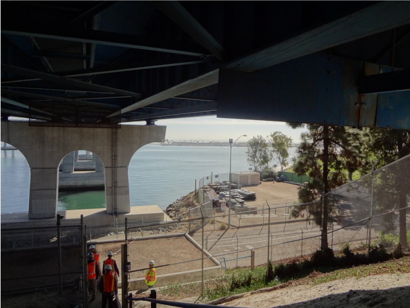
Figure 13 – Caltrans Maintenance Yard Connection Site Photo
