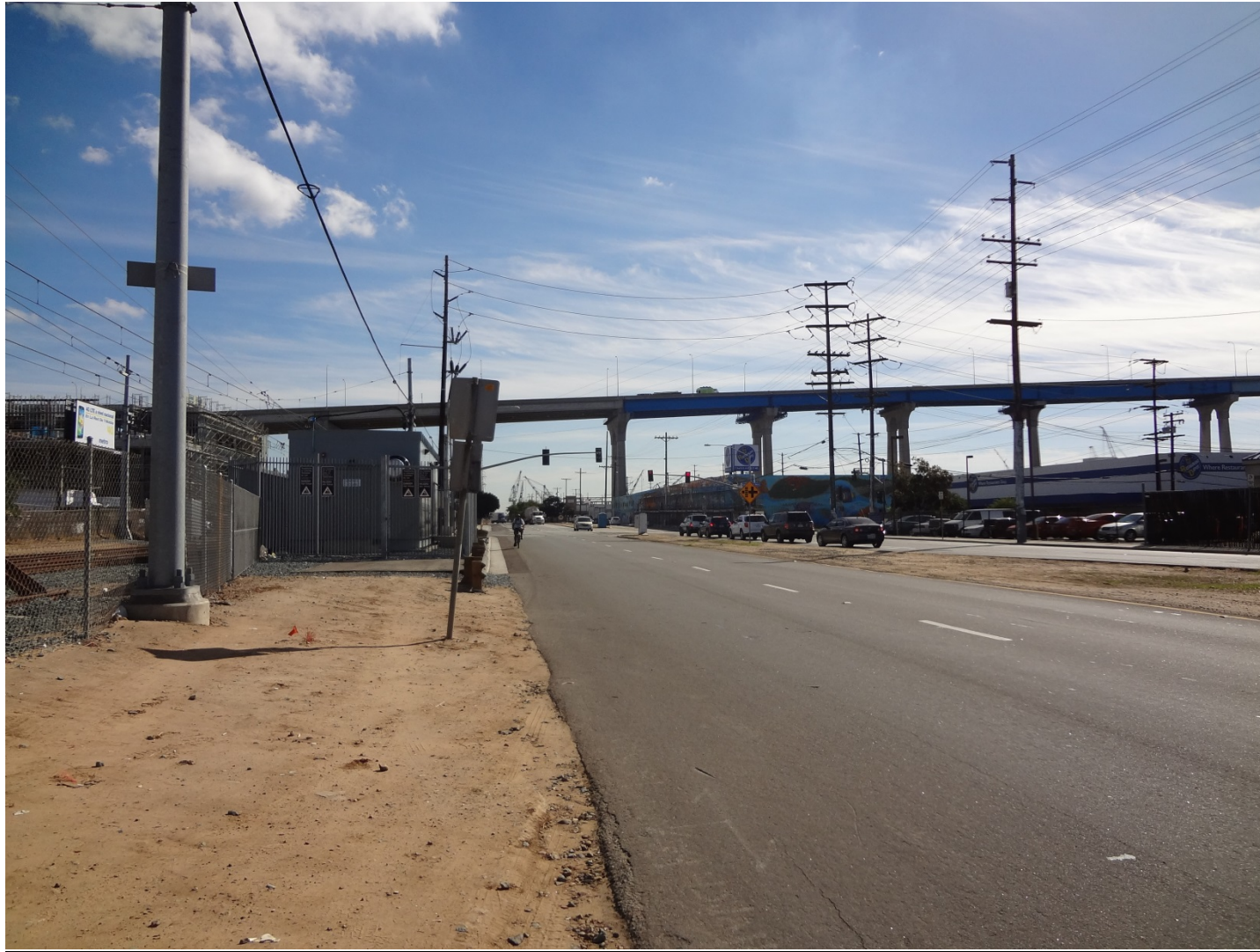
Figure 18 – Harbor Drive North Connection Point near Beardsley Street Site Photo
